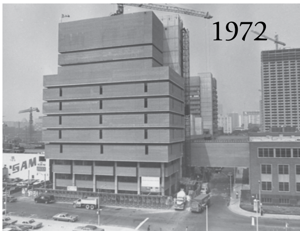
Photograph of the construction of the Library building circa 1972. The Sam the Record Man building is visible on the far left of the picture – the site for Ryerson's new Student Learning Centre. Courtesy of the Ryerson Archives
